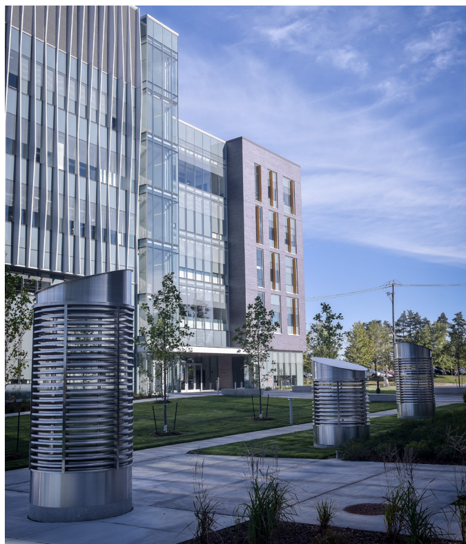
UTSC Environmental Science and Chemistry Building Earth Tubes
